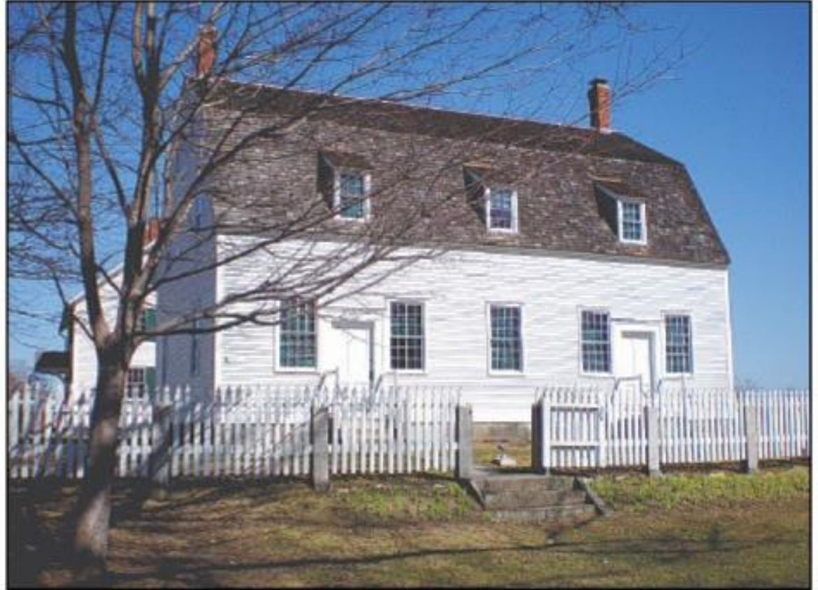
The Meetinghouse is located at Canterbury Shaker Village. It was built in 1792.
